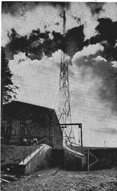
One of the aerial towers of the new 220 kw. Lahti, Finland, station is shown here. This is a long wave station on 1806 meters or 166 kcs.
